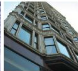
Reliance Building, Burnham and Root - early curtain wall framing
