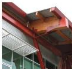
National Works Yard, Vancouver, LEED Gold
