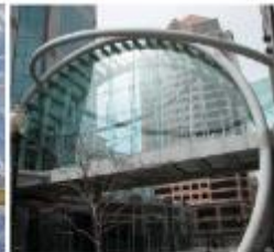
Pedestrian Bridge, Salt Lake City
